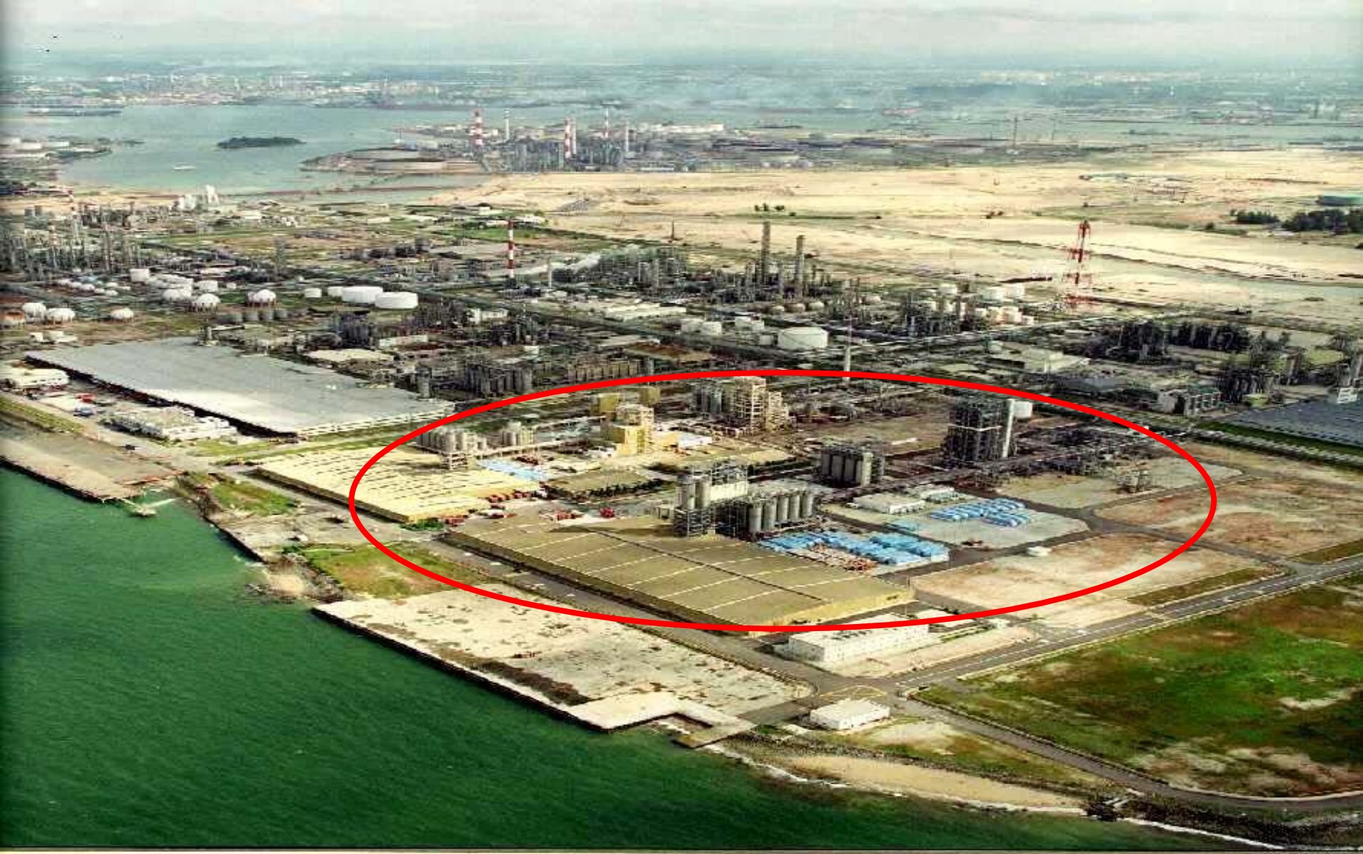
HDPE Plant located on Jurong Island, Singapore
